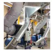
The customer decided to install Robox Screw in order to provide a curtain of air bubbles to prevent floating and submerged objects from entering the docking area. They
