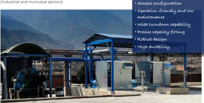
Modern wastewater treatment requires the movement of large volumes of air at low pressure and Robuschi's PD blower range provides a reliable source of air for its different processes.
